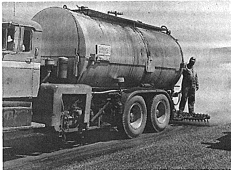
■ HOT kerosene-diluted asphalt-rubber mix is applied under pressure to existing surface. Then, precoated ¾ inch stone chips are spread at rate of 38 pounds/square yard. Daily production averaged 70,000 square yards.
