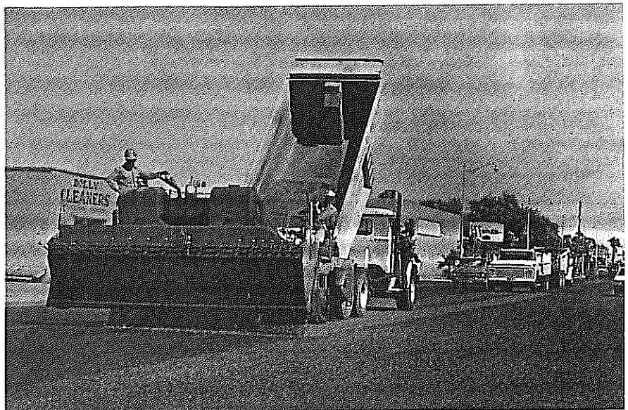
■ HOT kerosene-diluted asphalt-rubber mix is applied under pressure to existing surface. Then, precoated ¾ inch stone chips are spread at rate of 38 pounds/square yard. Daily production averaged 70,000 square yards.
