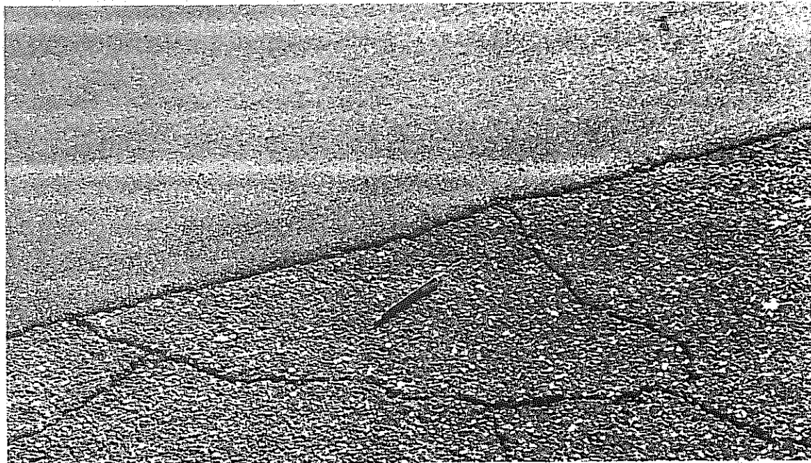
■ PLACED in 1969, asphalt-rubber shows no sign of reflective cracking, although the adjacent surface is badly cracked. Asphalt-rubber seal coats will reduce loss of curb depth, an inevitable effect of repeated overlaying.
