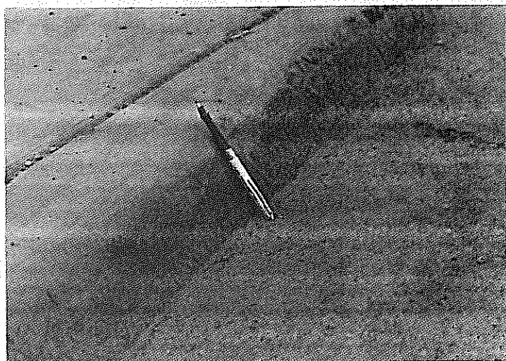
■ PLACED in 1969, asphalt-rubber shows no sign of reflective cracking, although the adjacent surface is badly cracked. Asphalt-rubber seal coats will reduce loss of curb depth, an inevitable effect of repeated overlaying.
