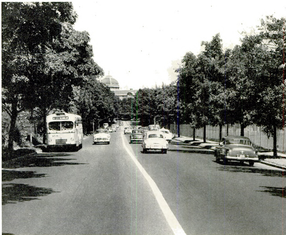
Asphalt-rubber surfaced street, Washington, D. C.
