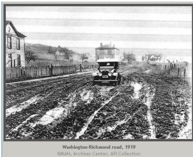
Figure 2 - Effect of too much water in the roadway (API 2005)
