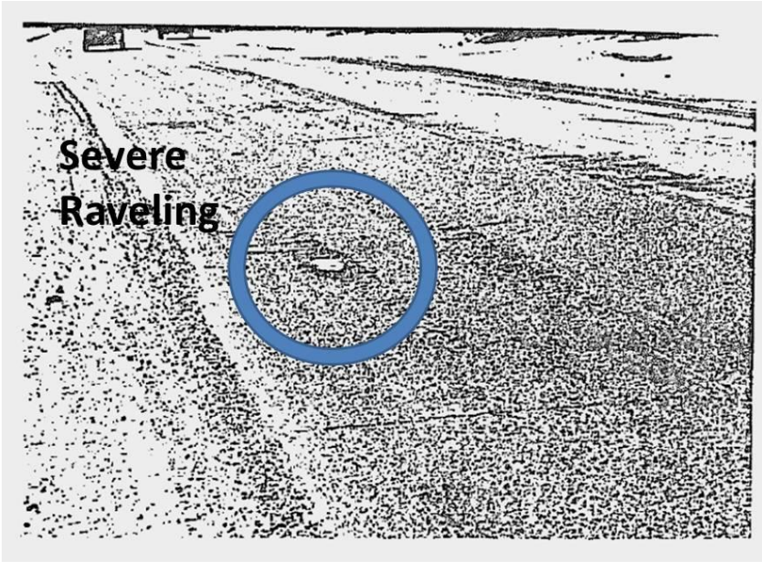
Figure 11 – Raveling of PLUS RIDE Mixture
