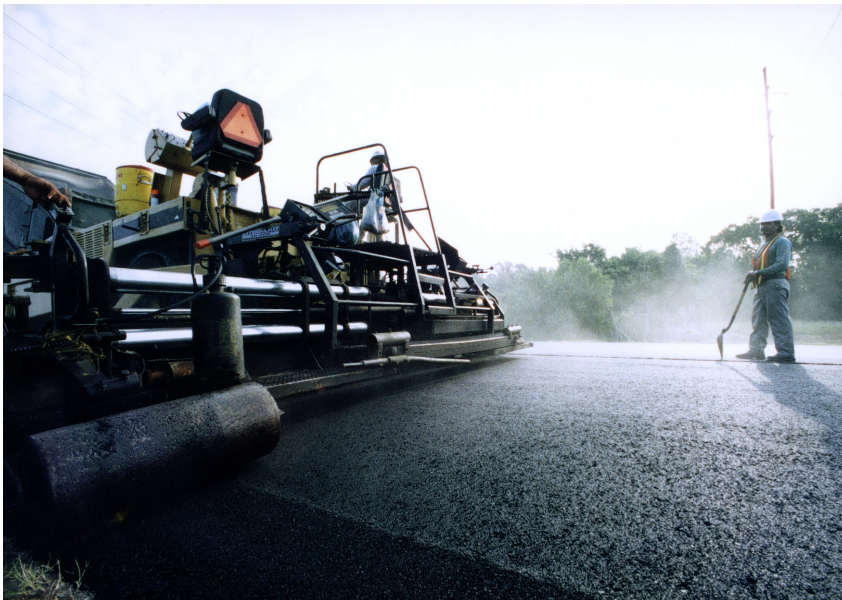
July 1998 placement of overlay on FM 2818.
