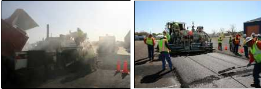
Figure 1. Comparison of hot- and warm-mix asphalt test track construction.
